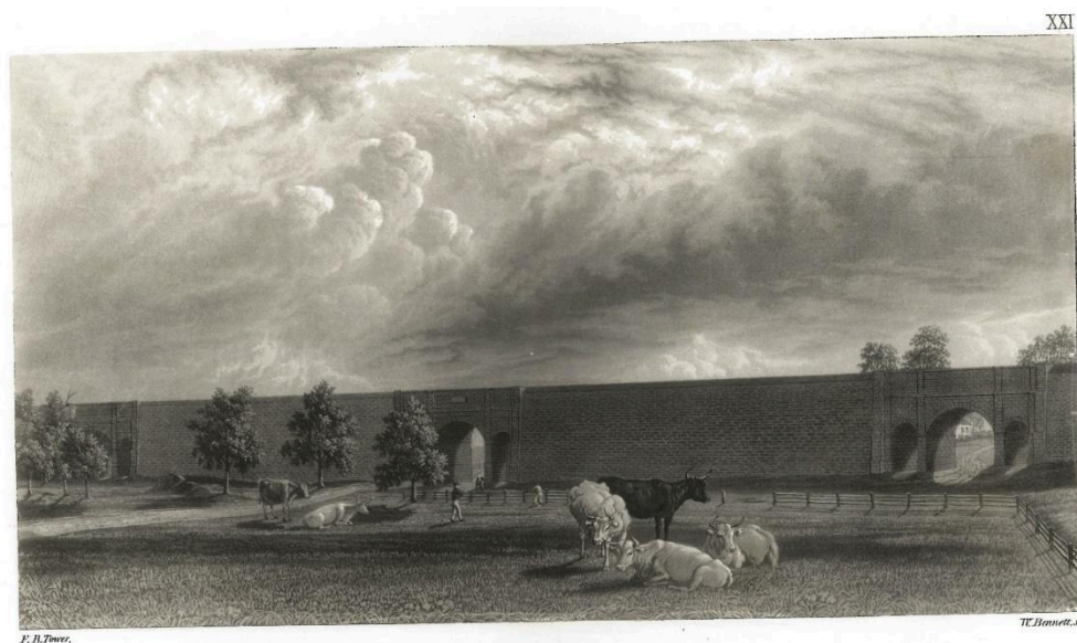
CROTON AQUEDUCT AT GLENDINNING VALLEY.
