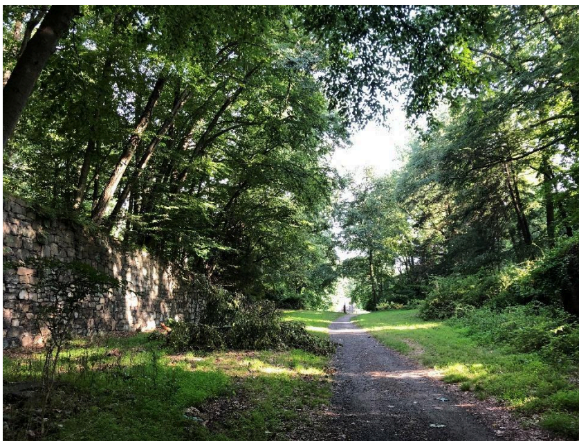
Figure 3. The aqueduct just North of Piping Rock Drive. 2
