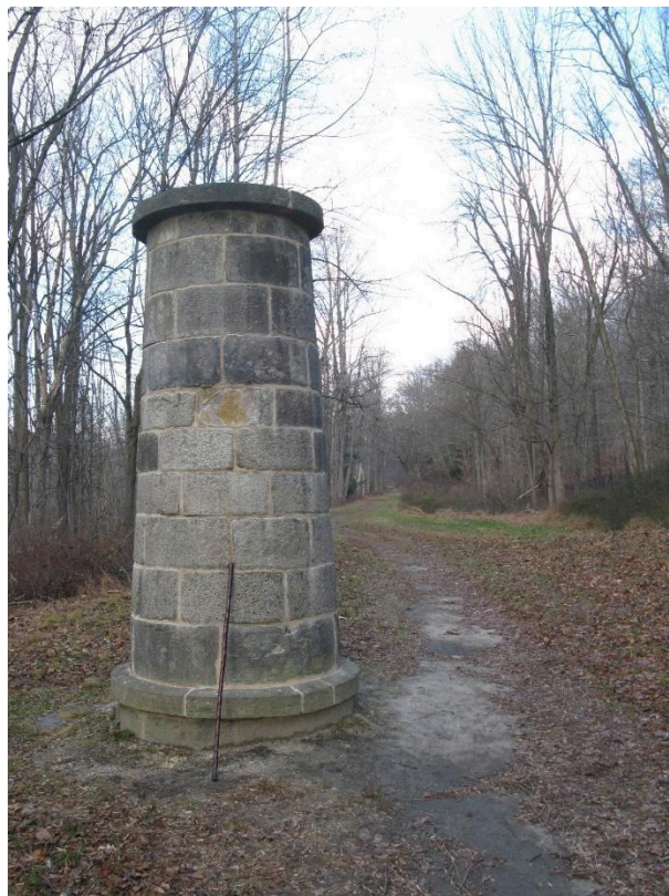
Figure 11. A ventilator shaft in autumn. 29
